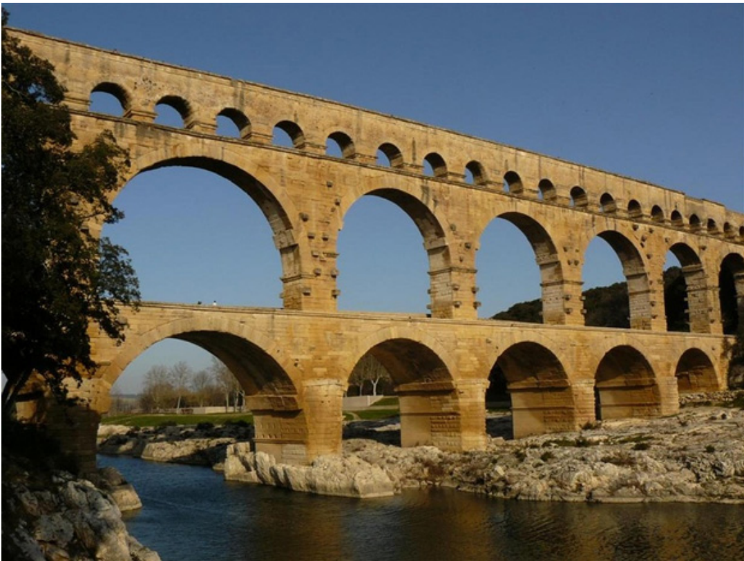
A Roman aqueduct
