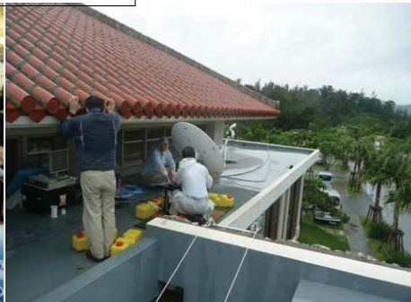
APEC展示で総務大臣や各国首脳に説明 万国津梁館屋上での可搬地球局設置作業 NICT Wireless Network Research Institute, National Institute of Information and Communications Technology
