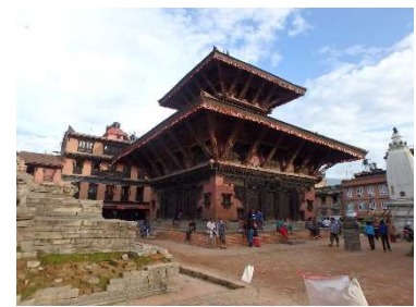
Fig. 3. Brick Masonry in Nepal
