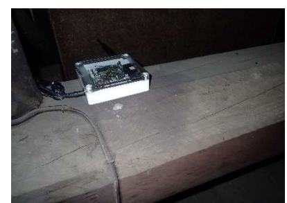
Fig. 6. Installation of Sensor
